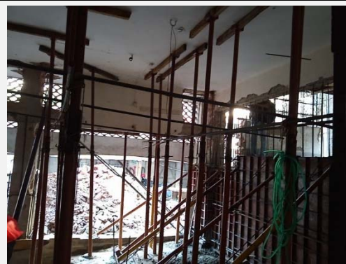
RC wall construction with supports
