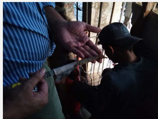
Quality control, checking the anchor hole
