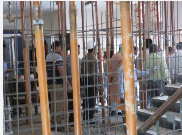
Actual Retrofitting work for site supervision
