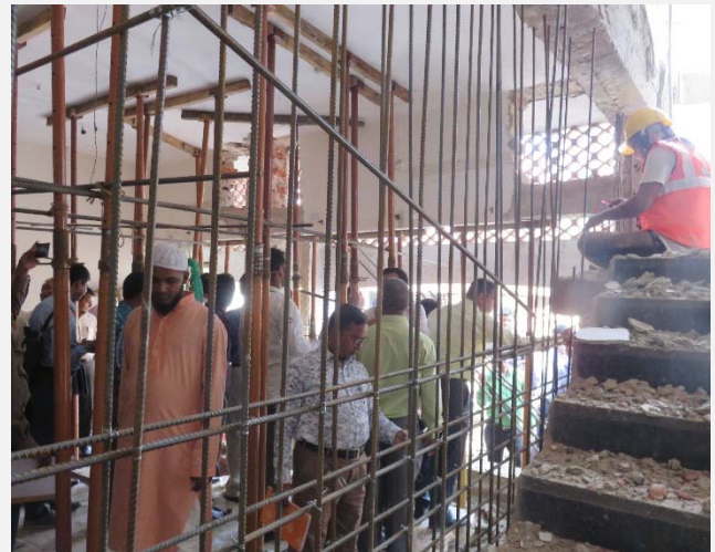
Retrofitting work site
